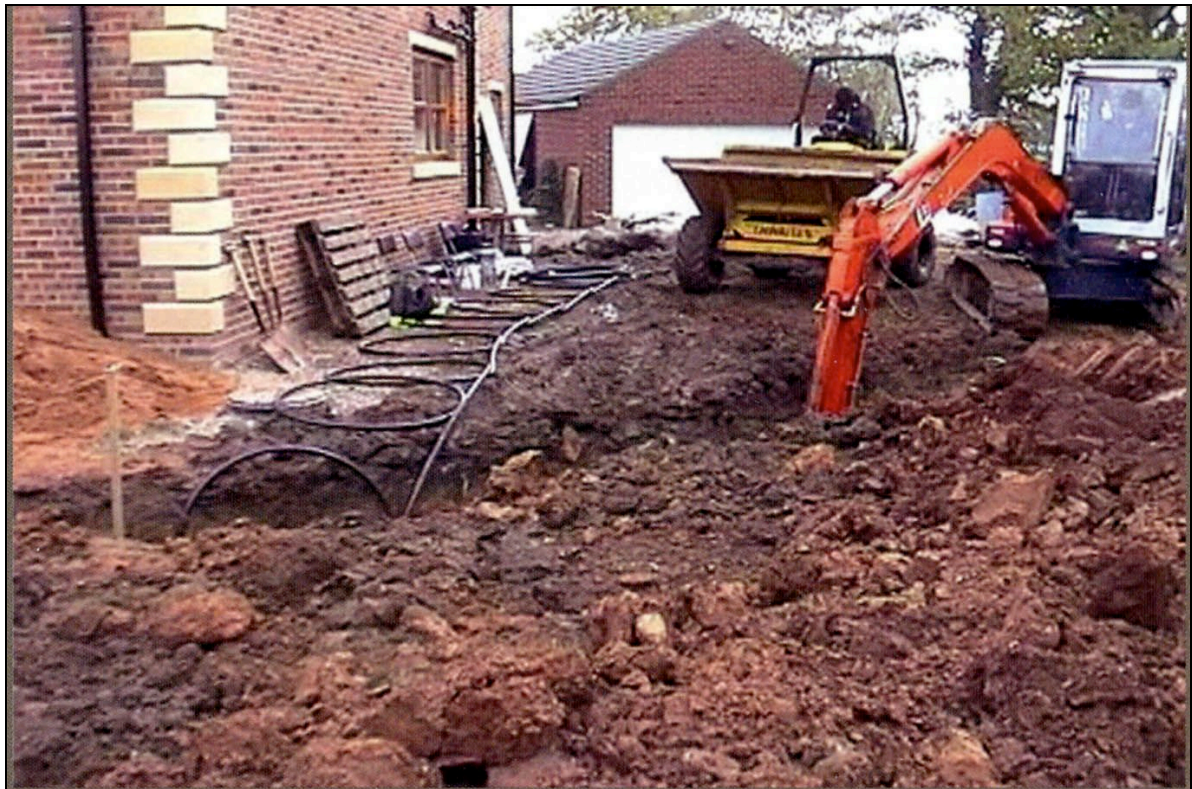
Preparation for ground loop
