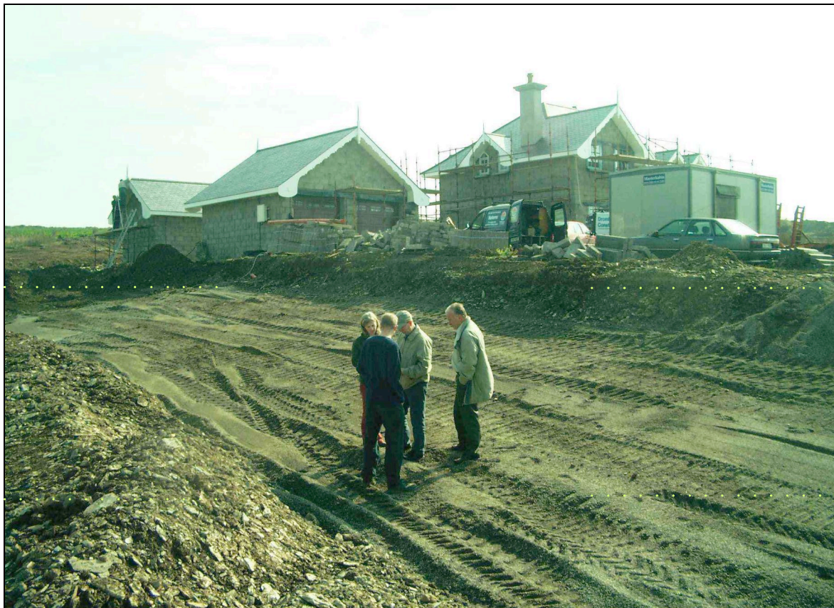
Collector site preparation
