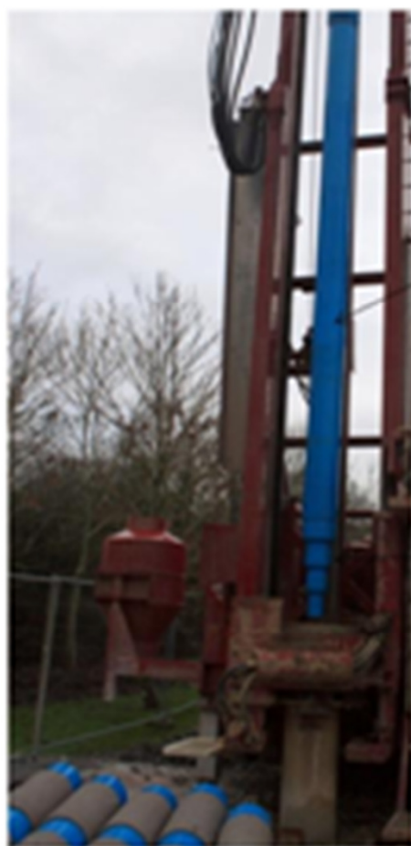
Installing Casing
