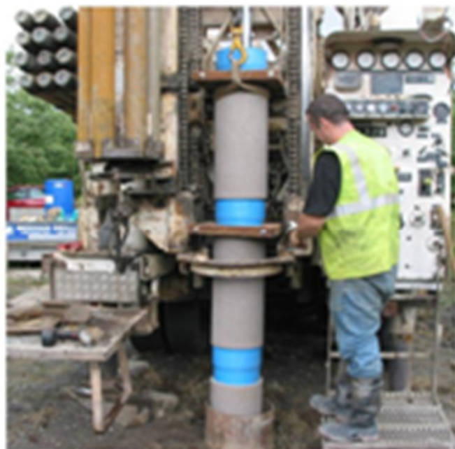
Installing Screen
