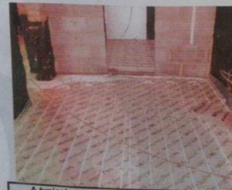
A typical standard Floor heating installation
